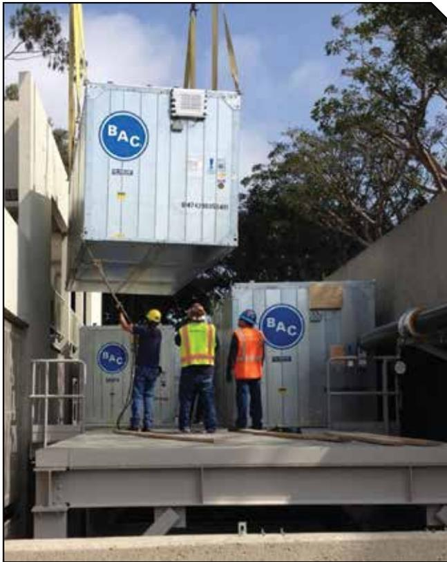
**FIGURE 3.** Due to city space restrictions, EMCOR Services Mesa Energy Systems came up with a solution to construct a brand new modular central plant (MCP) to house the chillers, pumps, VFDs, and DDC system in Molina Center's loading dock area.
