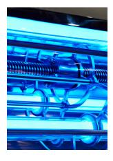
Another common technology leveraged to improve IAQ is ultraviolet C (UV-C) irradiation. Placed on the backside of cooling coils or in ductwork, UV-C bulbs offer continuous 24/7 protection from the buildup of pathogens
